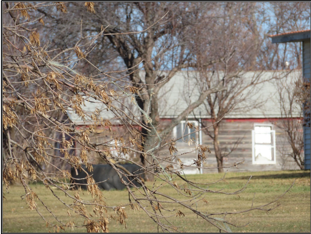
Figure B-5. Site 1: Outbuilding, south elevation, facing north.
