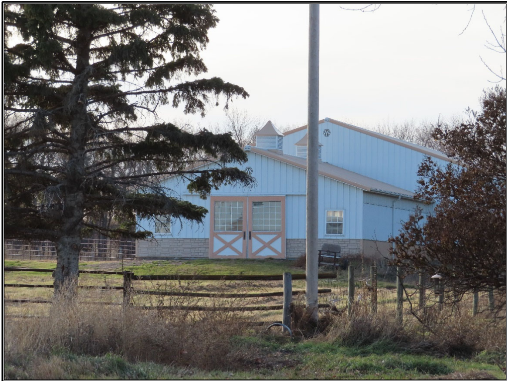
Figure B-64. Site 9: Barn No. 3, east and north elevations, facing west-southwest.
