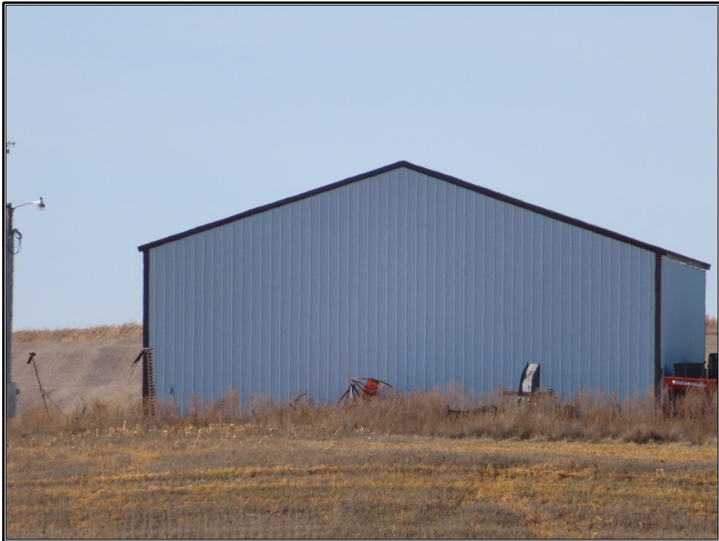
Figure B-34. Site 5: Metal building, east elevation, facing west.
