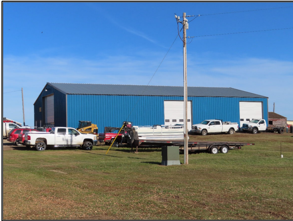
Figure B-9. Site 1: Metal building, south and west elevations, facing northeast.
