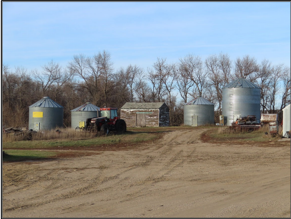
Figure B-51. Site 8: Grain bins and outbuilding, south and east elevations, facing northwest.
