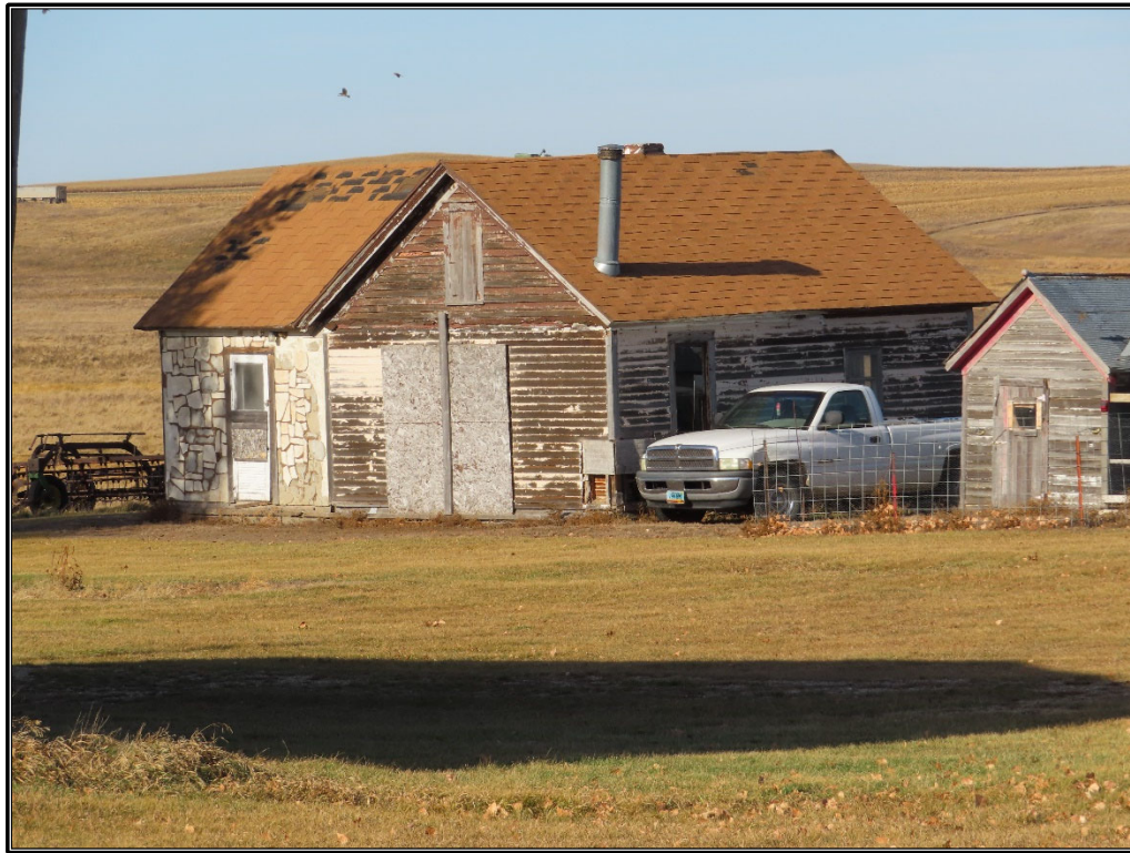
Figure B-21. Site 3: Façade (east) and south elevations of second residence, facing northwest.
