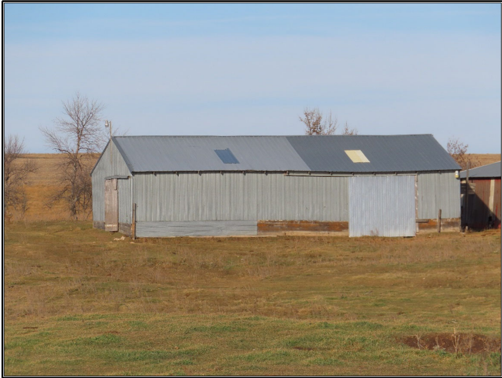
Figure B-41. Site 6: Metal building No. 2, south and west elevations, facing northeast.
