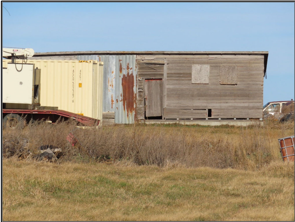
Figure B-14. Site 1: Outbuilding, south elevation, facing north.
