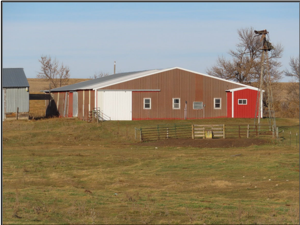
Figure B-42. Site 6: Metal building No. 3, south and west elevations, facing northeast.
