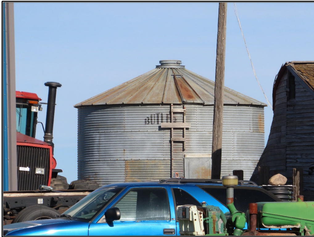
Figure B-11. Site 1: Grain bin, facing northwest.
