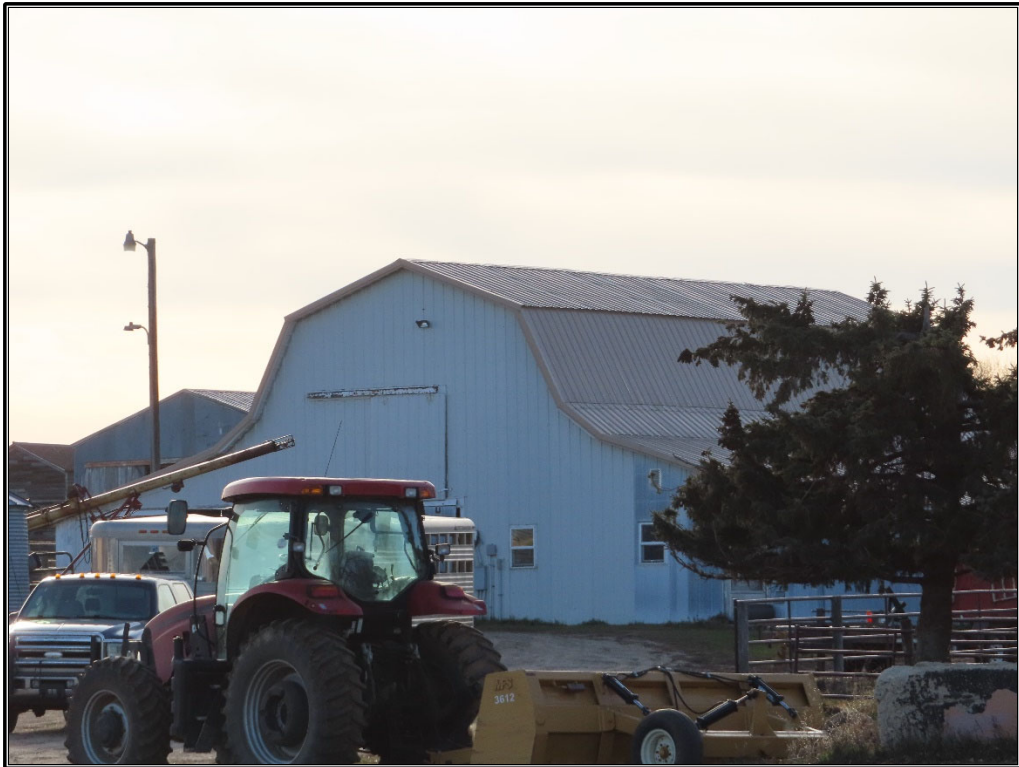
Figure B-62. Site 9: Barn No. 2, east and north elevations, facing southwest.
