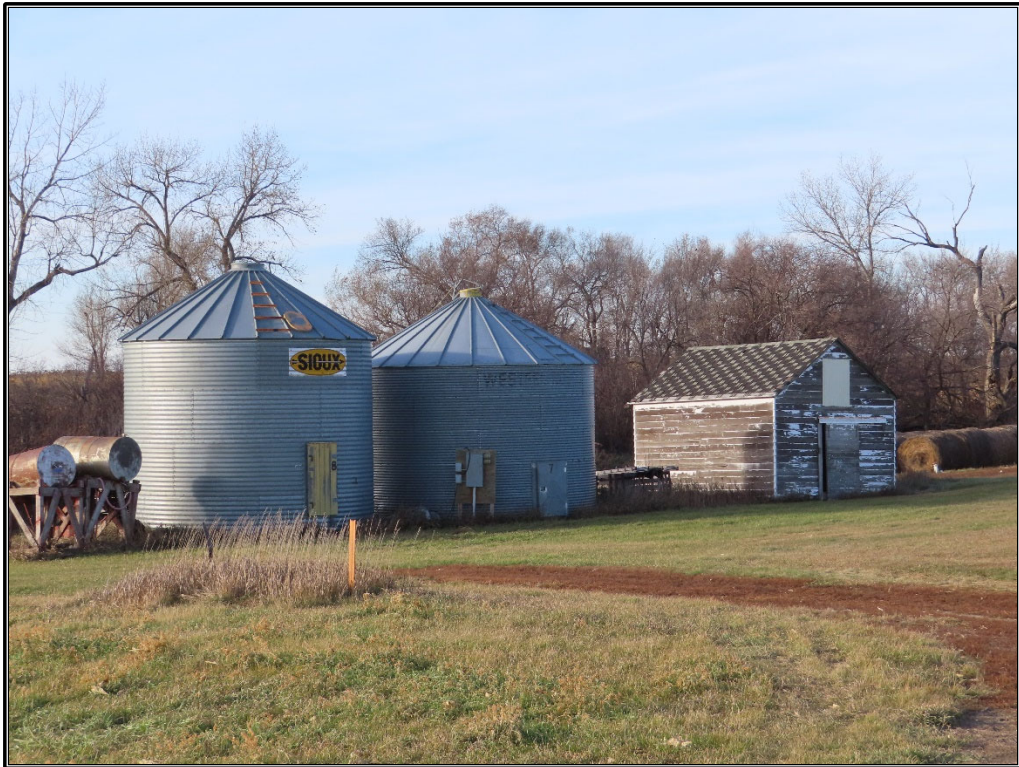
Figure B-50. Site 8: Grain bins and garage, south and east elevations, facing northwest.
