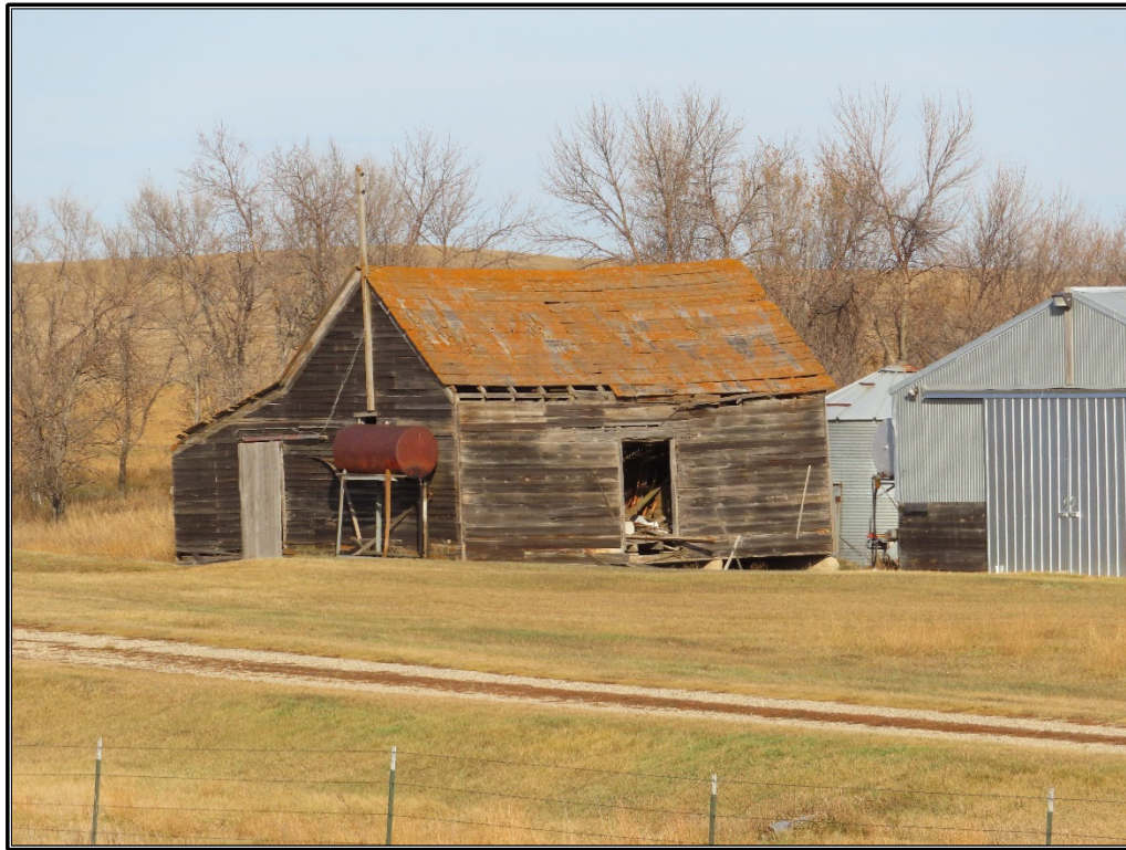
Figure B-39. Site 6: Barn, south and west elevations, facing northeast.
