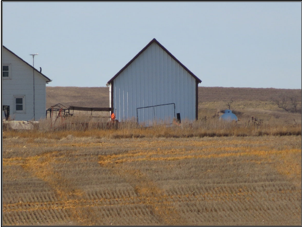
Figure B-35. Site 5: Outbuilding, east elevation, facing west.
