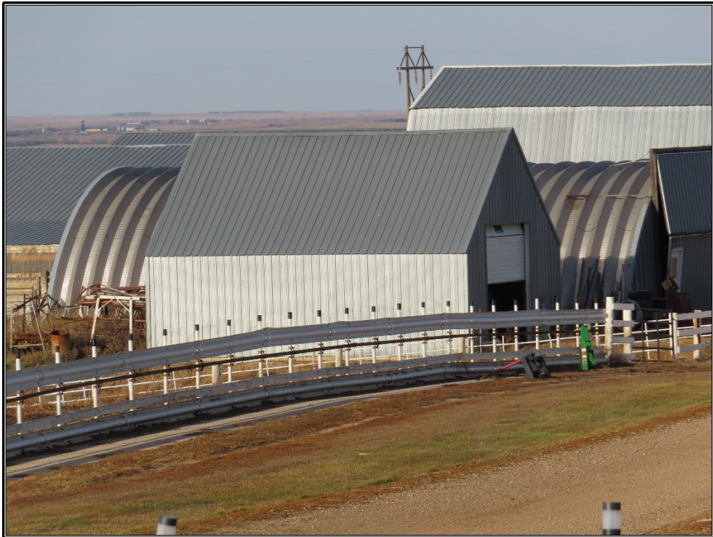
Figure B-46. Site 7: Garage, east and south elevations, facing northwest.
