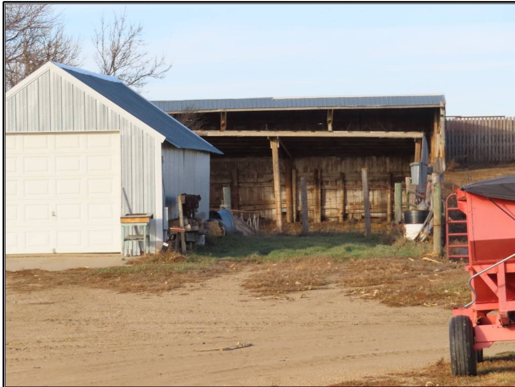
Figure B-54. Site 8: Animal shelter, south elevation, facing north.
