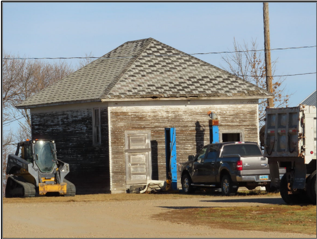
Figure B-6. Site 1: Garage, south and west elevations, facing north-northeast.
