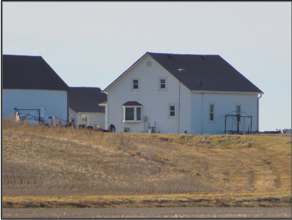
Figure B-31. Site 5: Façade (east) and north elevation, facing southwest.
