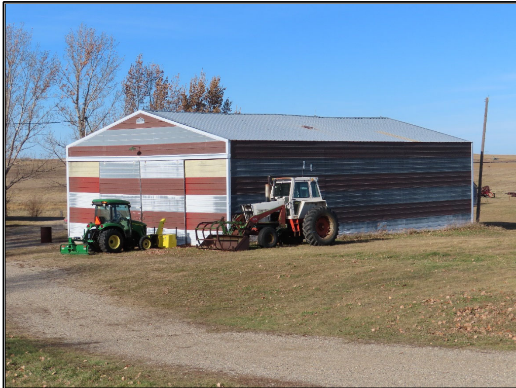
Figure B-22. Site 3: Metal outbuilding, south and east elevations, facing northwest.
