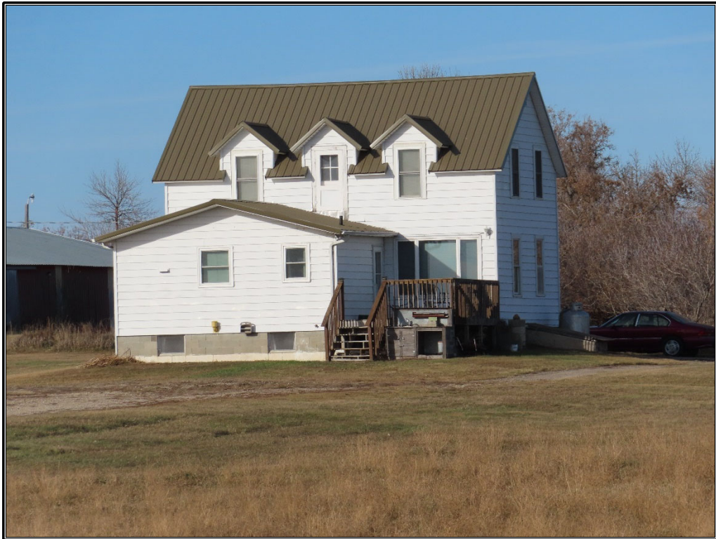
Figure B-36. Site 6: Façade (south) and east elevations of the residence, facing northwest.
