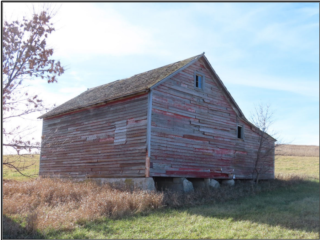
Figure B-26. Site 4: East and north elevations of residence, facing southwest.
