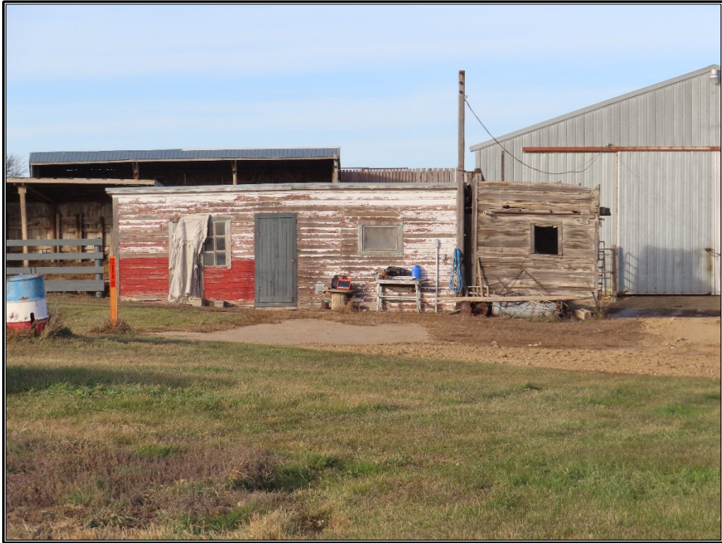
Figure B-55. Site 8: Outbuilding, south and east elevations, facing northwest.
