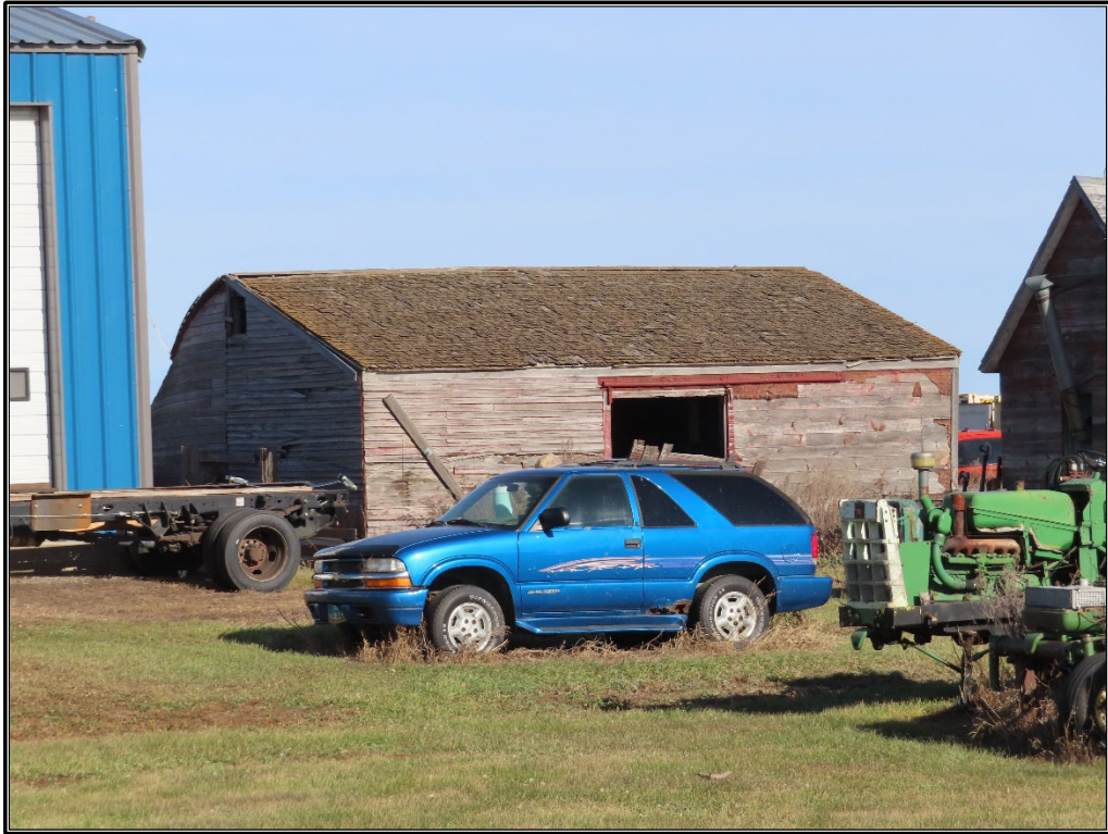
Figure B-13. Site 1: Small barn, west and south elevations, facing northeast.
