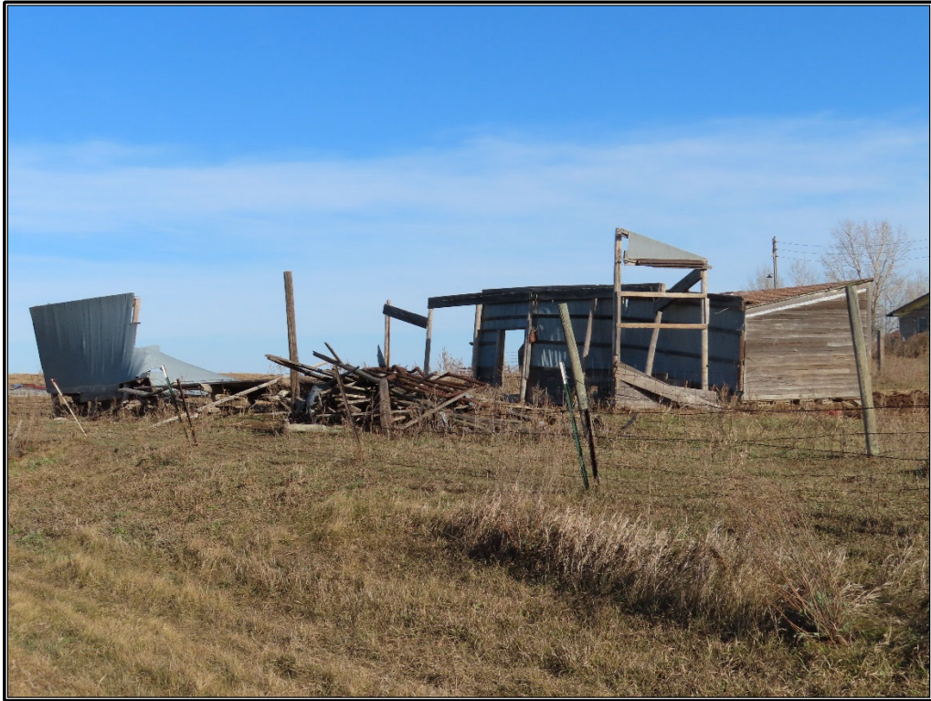
Figure B-19. Site 2: Animal shelter and outbuilding ruin, south and west elevations, facing northeast.
