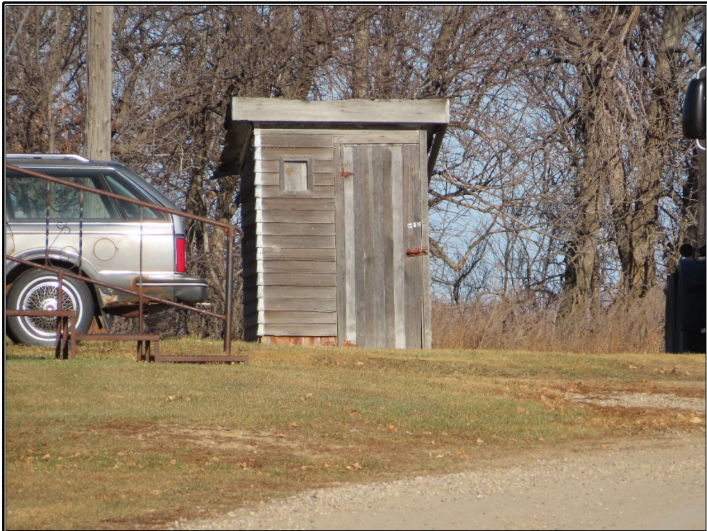
Figure B-4. Site 1: Privy, facing north.
