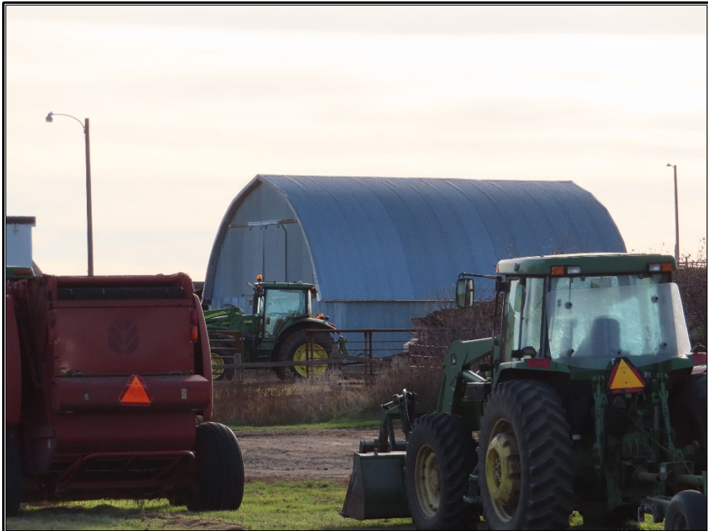
Figure B-60. Site 9: Barn No. 1, north and east elevations, facing southwest.
