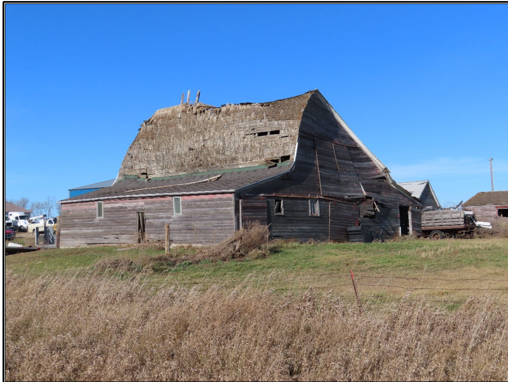
Figure B-10. Site 1: Barn No. 2, south and east elevations, facing northwest.
