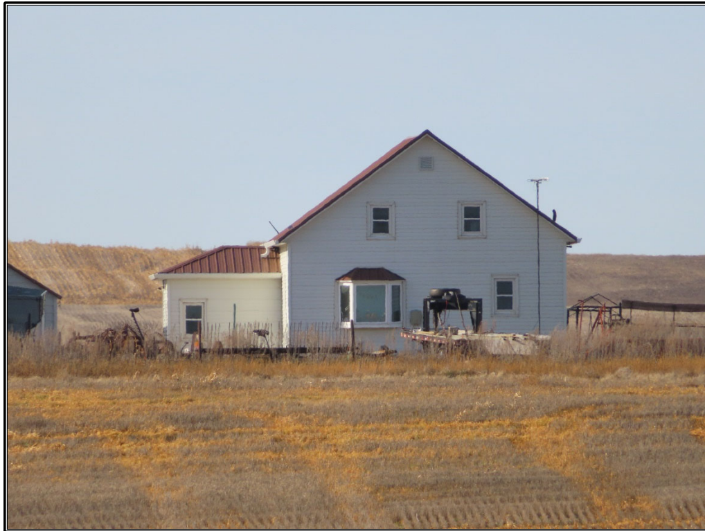
Figure B-30. Site 5: Façade (east elevation) of the residence, facing west.
