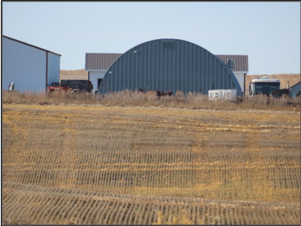
Figure B-33. Site 5: Quonset hut, east elevation, facing west.
