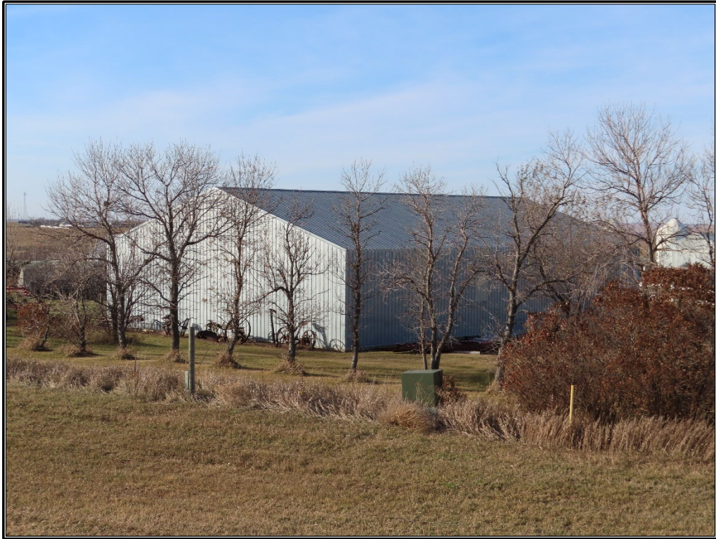
Figure B-49. Site 7: Metal building, south and east elevations, facing northwest.
