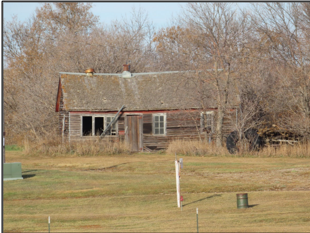
Figure B-38. Site 6: Outbuilding, south elevation, facing north.
