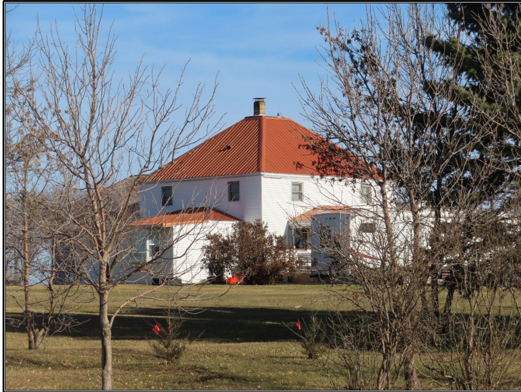
Figure B-1. Site 1: Façade (south) and east elevations of residence, facing northwest.
