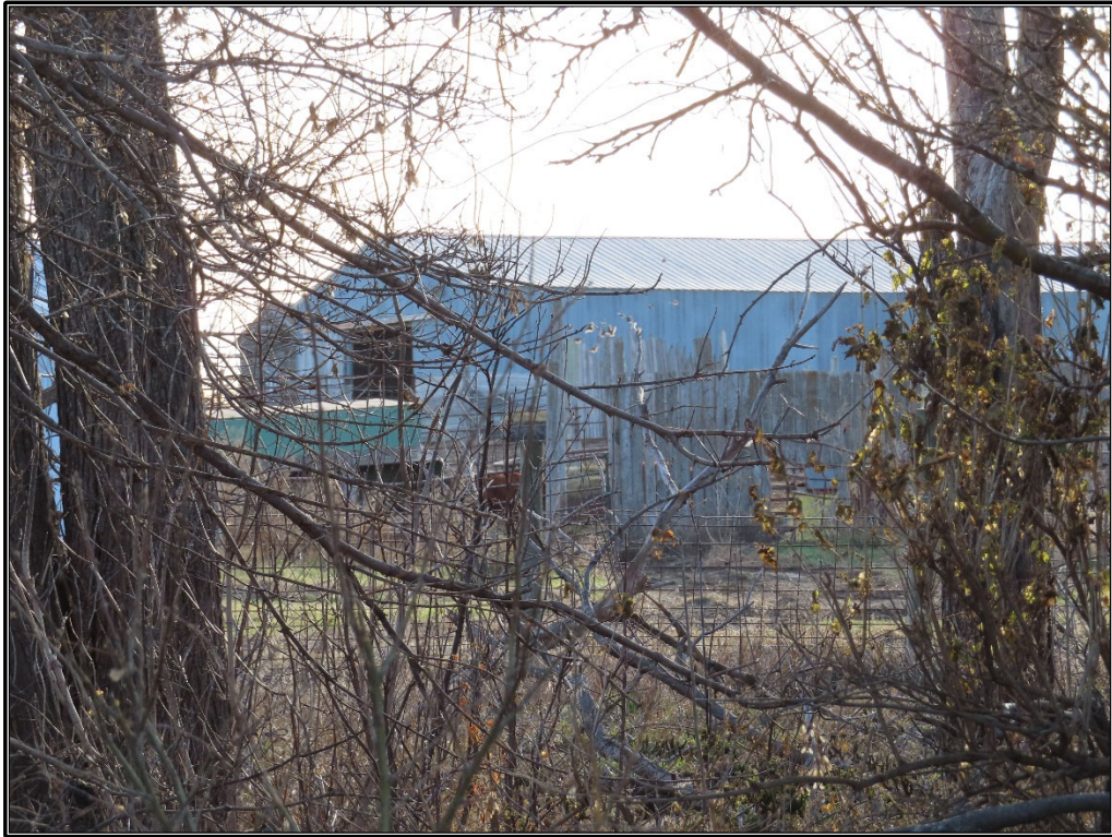
Figure B-63. Site 9: Metal building, east and north elevations, facing southwest.
