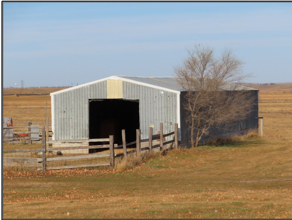
Figure B-23. Site 3: Metal outbuilding, south and east elevations, facing northwest.
