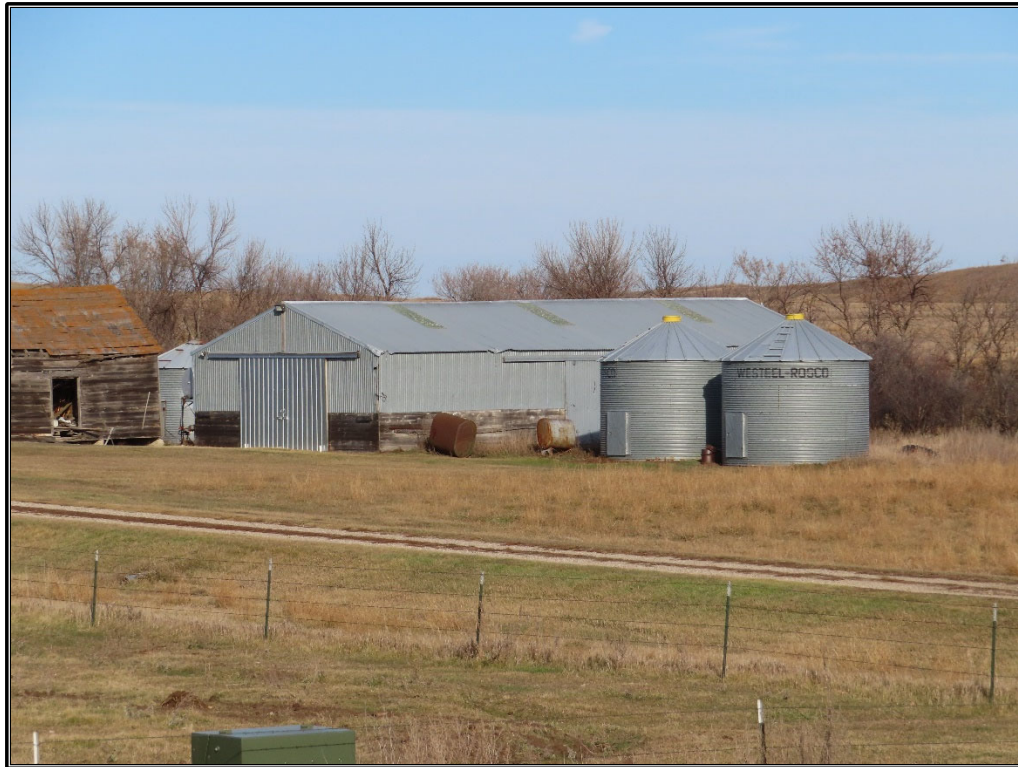
Figure B-40. Site 6: Metal building and grain bins, south and west elevations, facing northeast.
