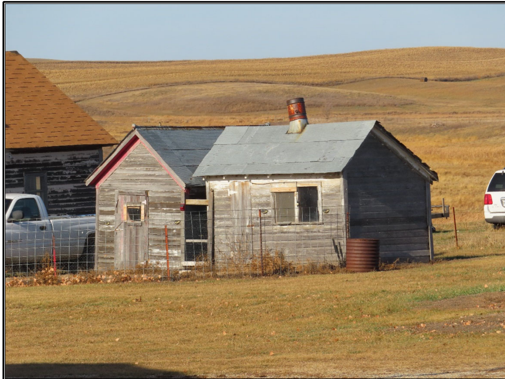
Figure B-24. Site 3: Outbuildings, south and east elevations, facing northwest.
