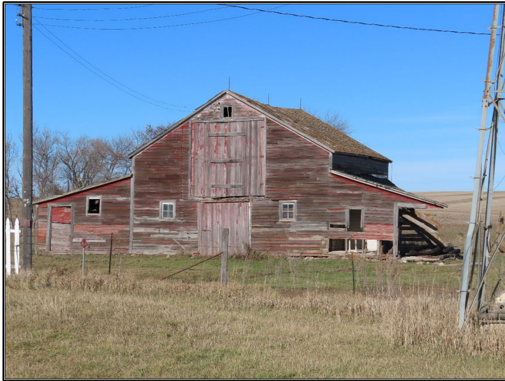
Figure B-27. Site 4: Barn, south elevation, facing north.
