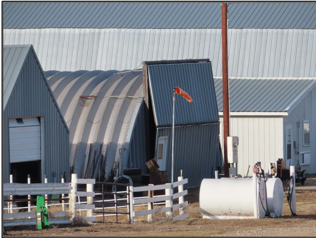
Figure B-47. Site 7: Quonset hut, east and south elevations, facing northwest.
