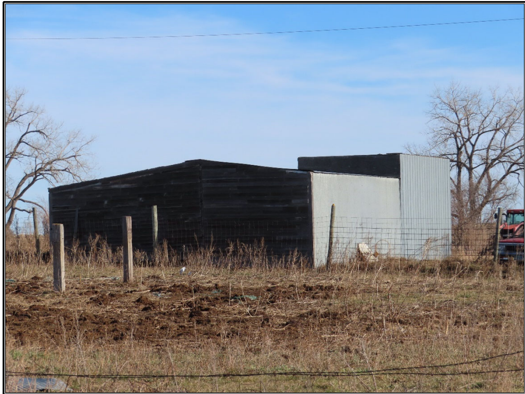
Figure B-18. Site 2: Metal outbuilding, south and west elevations, facing northeast.
