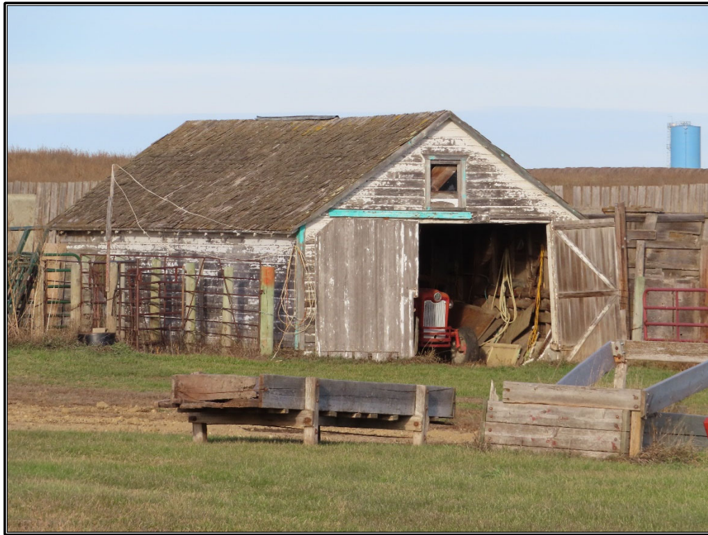
Figure B-53. Site 8: Garage No. 2, west and south elevations, facing northeast.
